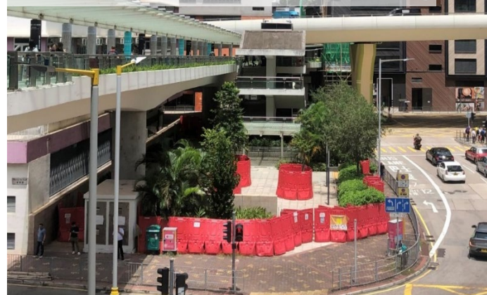
Improvement of Nam Long Shan Road SoA 改善南朗山道休憩處
