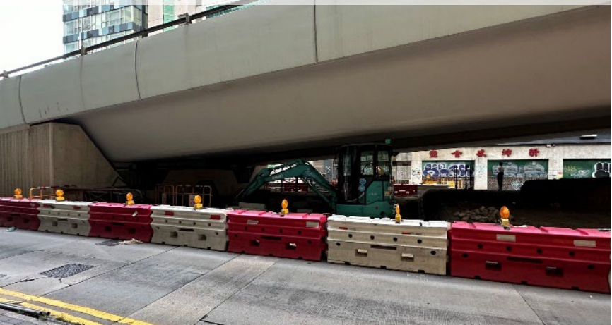
Widening of footpaths along WCH Road adjoining Ocean Park Plant Nursery 擴闊黃竹坑道近海洋公園苗圃的行人路
