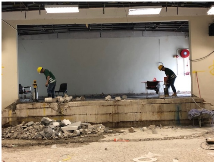
重置職員更衣室 Re-provision of staff changing rooms
