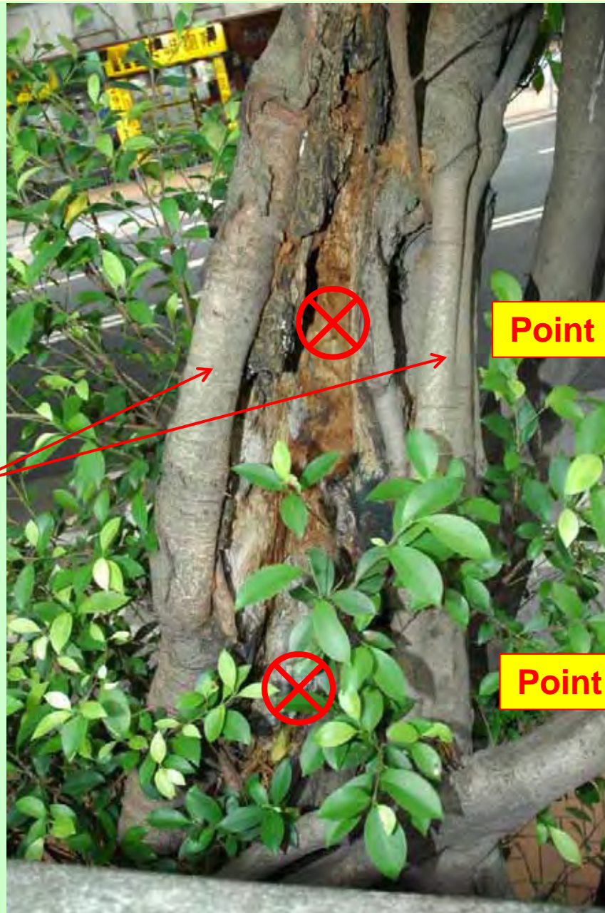
Photo T5-8. Large cavity with decay extending from trunk base upwards. Crosses denote drilling positions.
