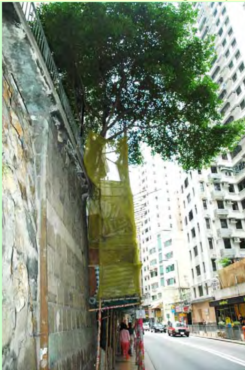
Photo T1-5. The young Chinese Banyan with a small crown hangs well above the carriageway.
