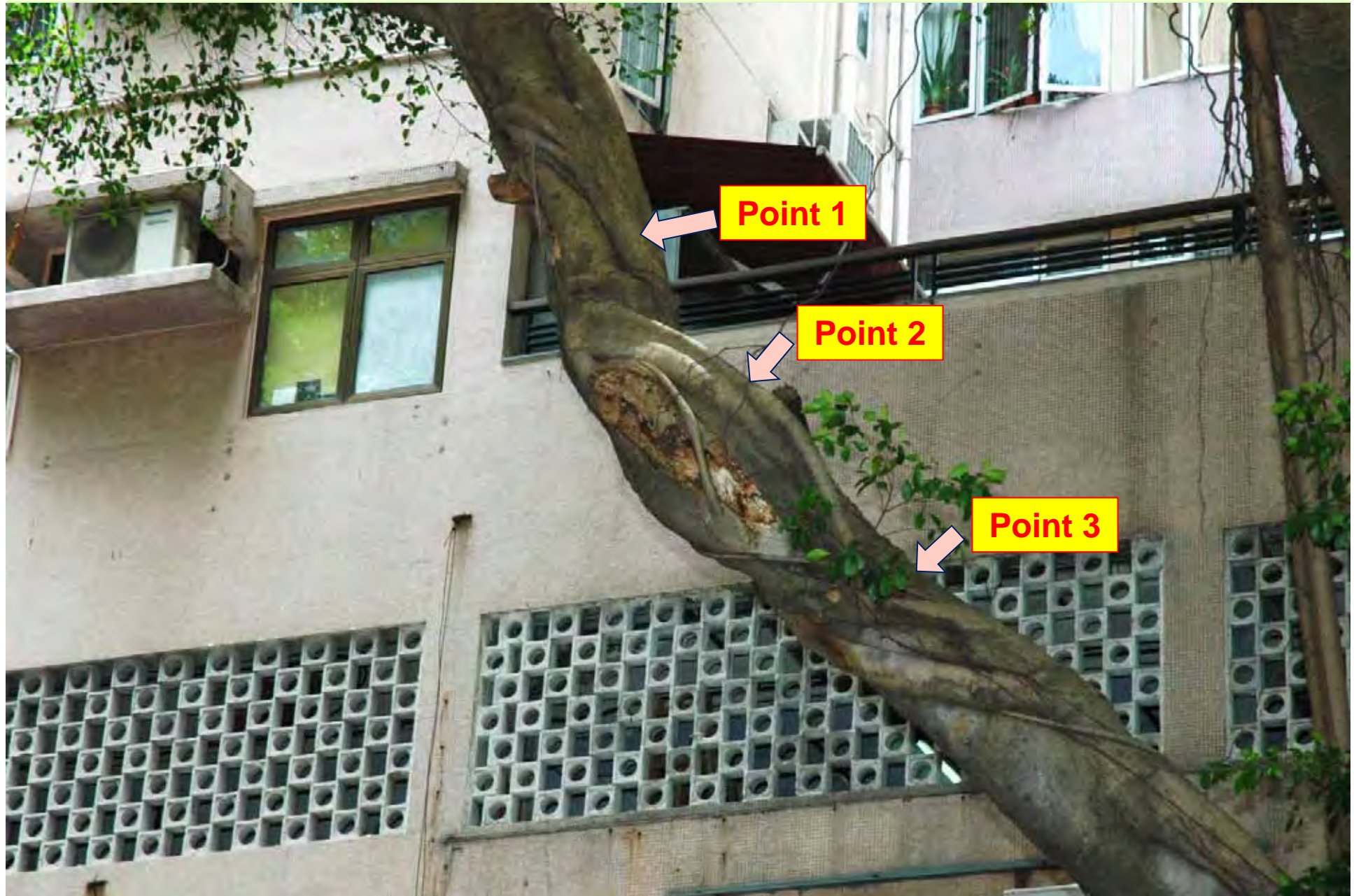
Photo T2-31. Stem A1 has a large wound with decay and bulgewood formation. Arrows indicate drilling positions.
