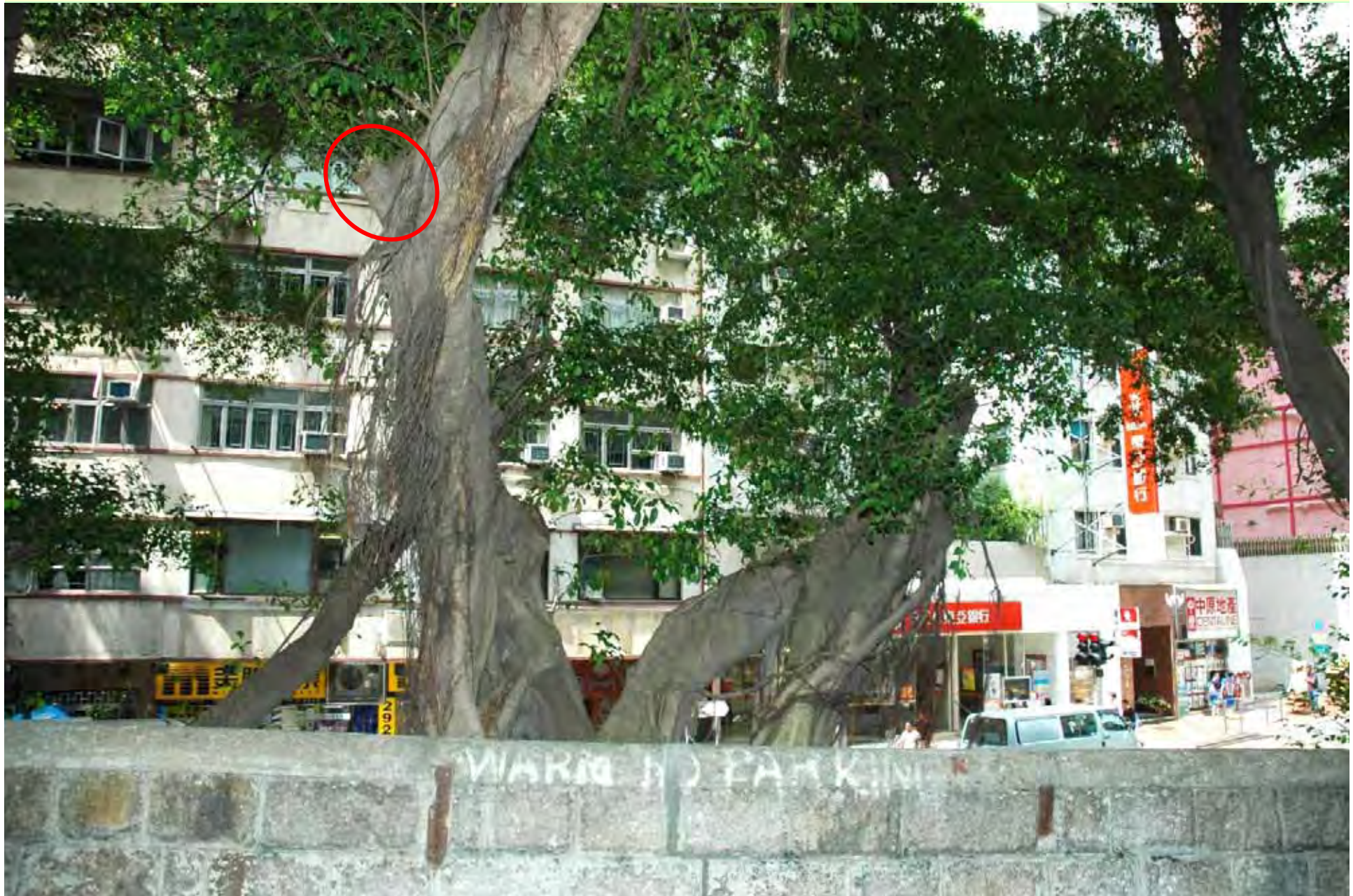
Photo T4-28. Branch stub of stem B with decay.
