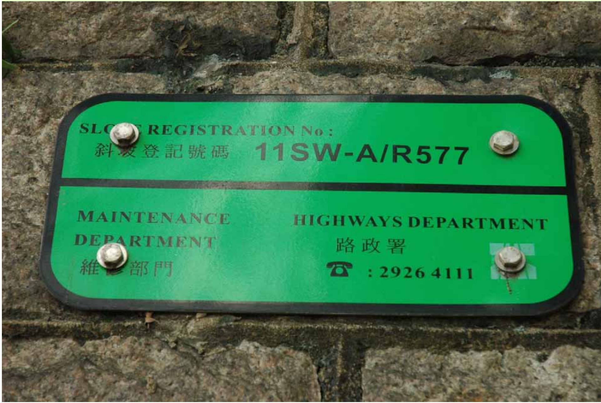
Photo T0-2. The old stone wall together with its stonewall trees are maintained by the Highways Department.
