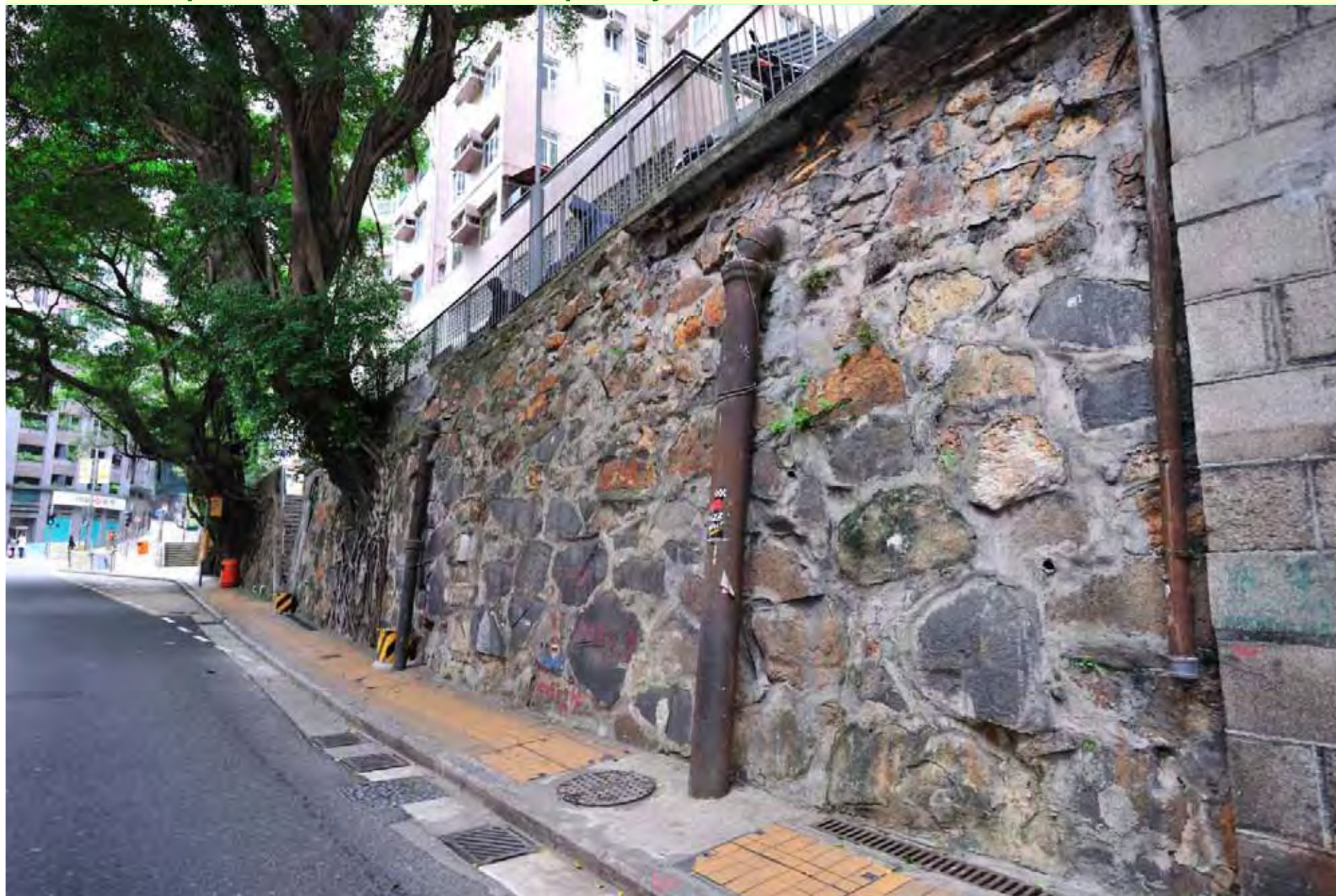
Photo T0-9. The stone wall viewed from the west, with irregularly shaped and sized and partly-weathered volcanic stones..
