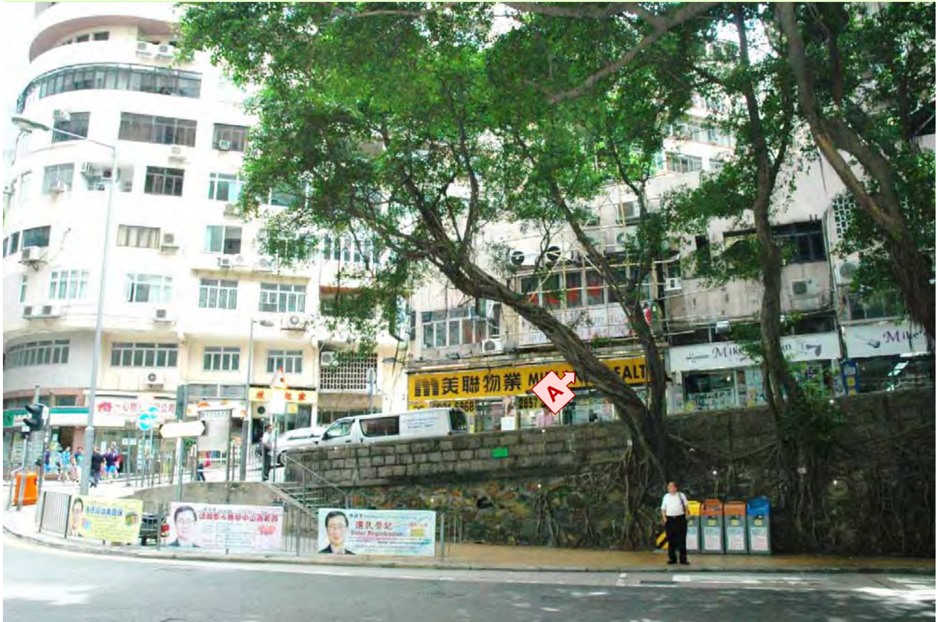
Photo T6-10. Stem A tilts notably towards the east.
