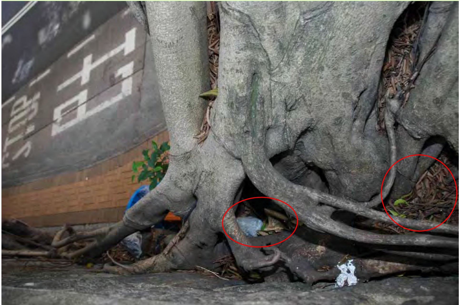
Photo T6-8. The organic litter and rubbish accumulated in the gap between the trunk and the wall can be regularly removed.
