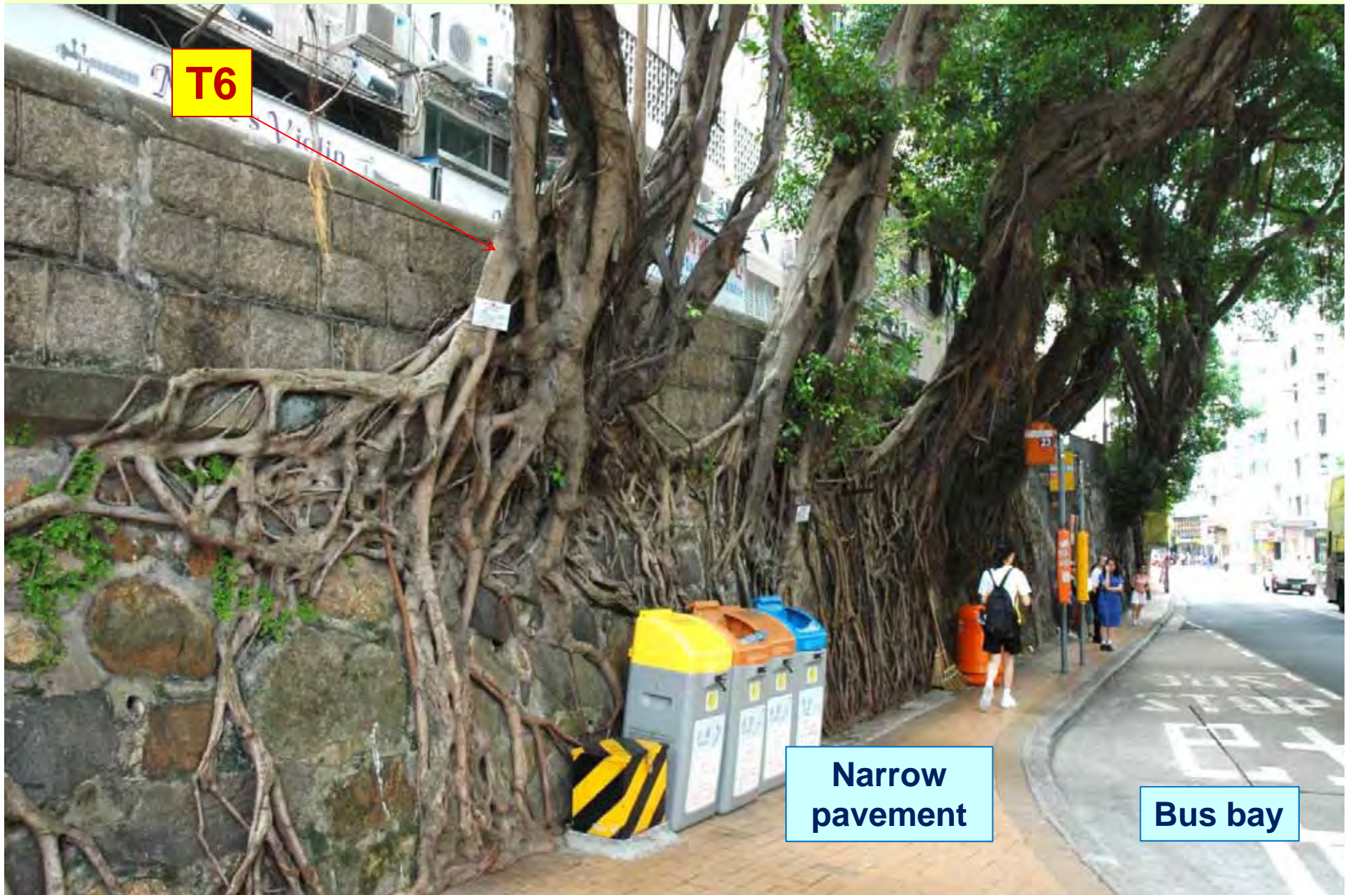
Photo T0-8. The old masonry wall viewed from the east, being shorter at the east side and taller towards the west.
