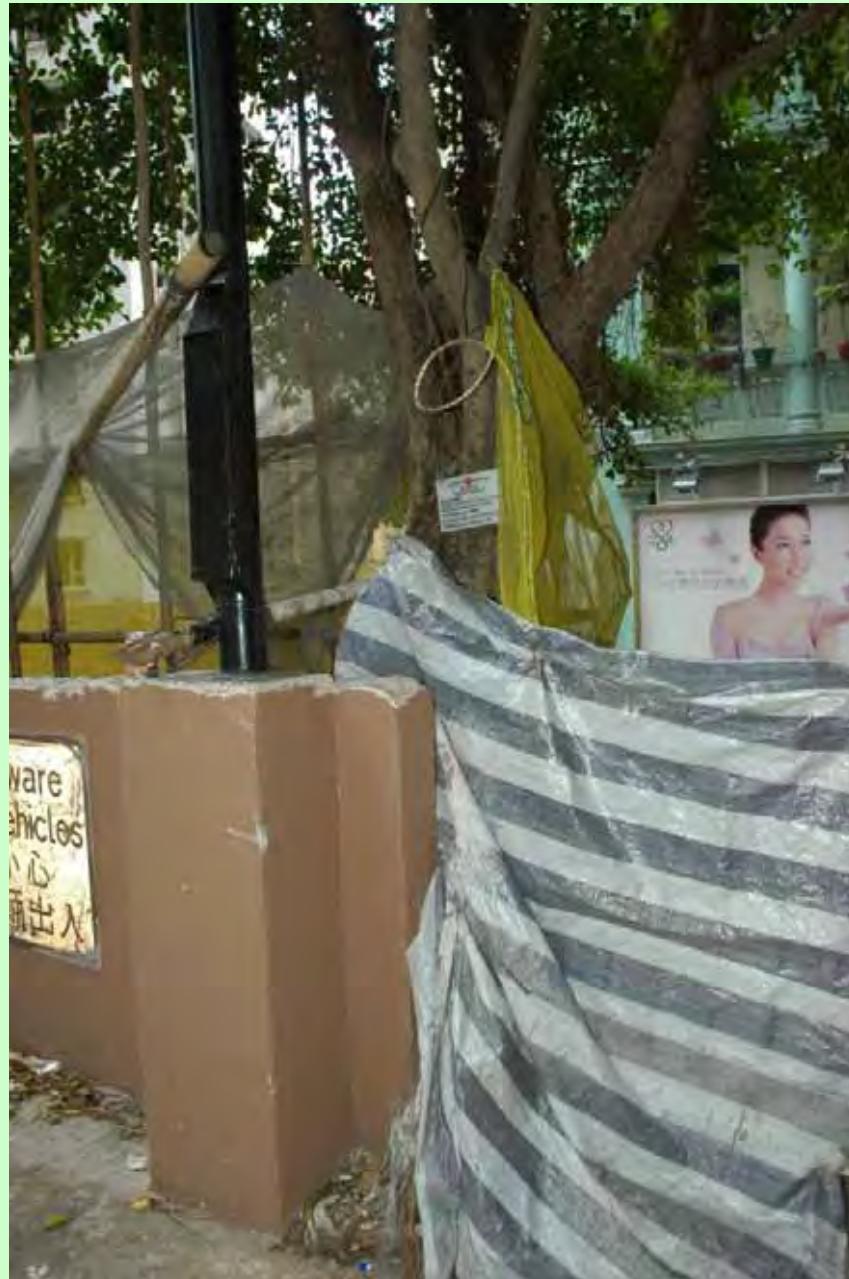
Photo T1-8. Renovation work at the adjacent building has used the tree to support its nylon net and sheet.
