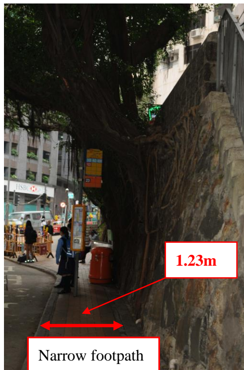
Photo 2.6 – Southern footpath at Bonham Road (viewing from the west)
