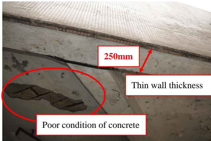
Photo 2.3 – Existing condition of nearby building
