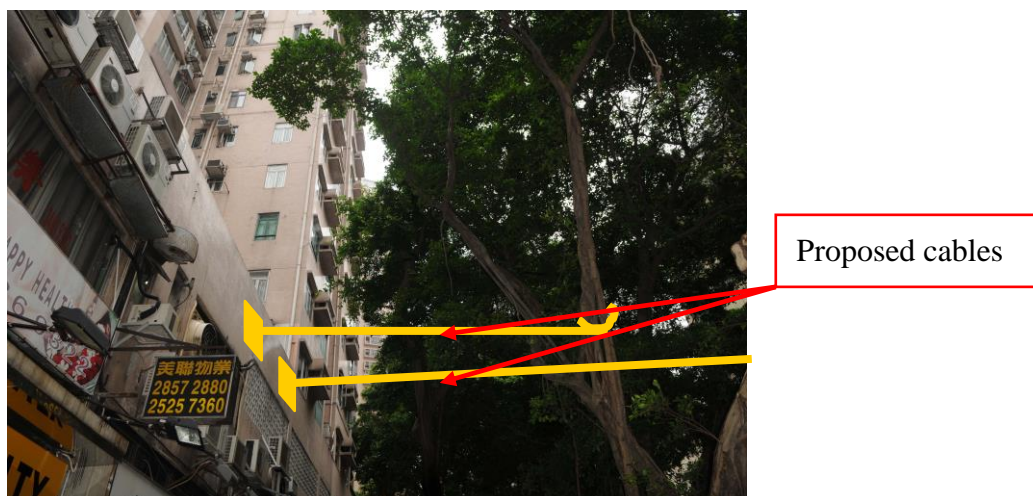
Photo 2.2 – Proposed cables anchor on the nearby building
